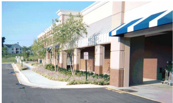
Example of Foundation Landscaping
