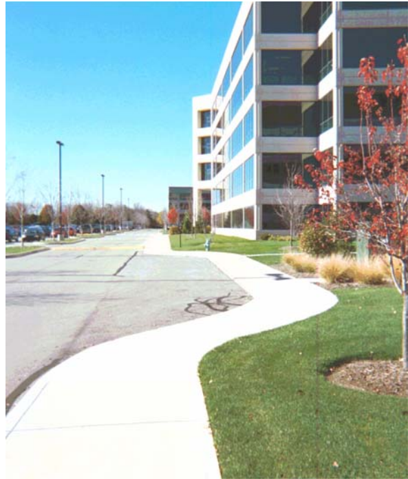
Pull-Off Loading Area
